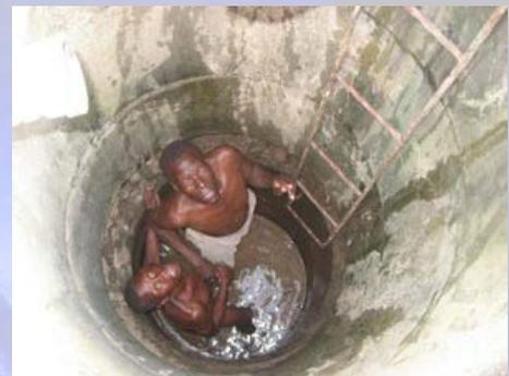
Well drilling consisted of 2 men in a three foot diameter hole scooping mud and water into buckets to be raised by ropes. As fast as they worked the water continued to fill the hole. This required the use of a broken water pump and petro to fuel the
